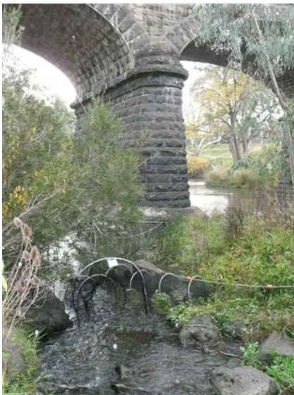
Macedon St Bridge, Apex Park Sunbury
